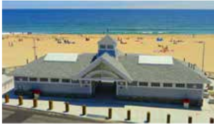
Marine Memorial & North Bathhouse
